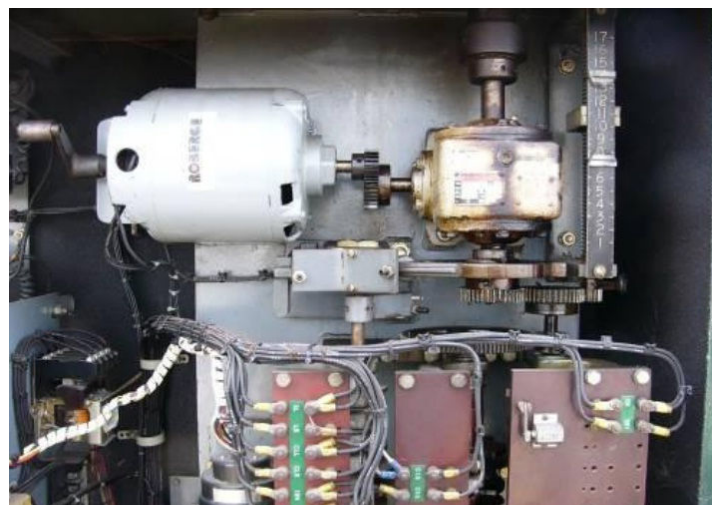
Figure 7. OLTC motor drive
