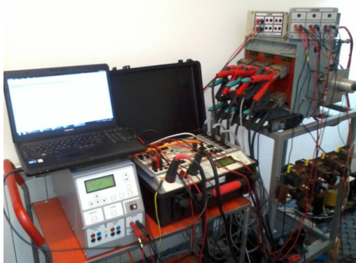
Figure 3.1 Timing tests on a circuit breaker
